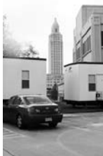
Following Hurricane Katrina, the Clerk of Court secured two trailers that served as the temporary office in Baton Rouge.
